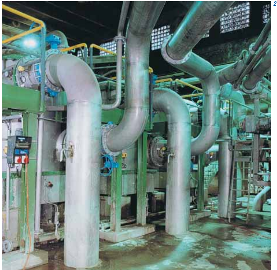
Fig. 2: Slotted fine screening system.
