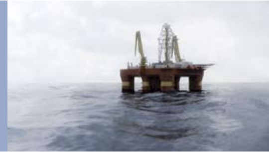
The Voith Radial Propellers keep floating offshore platforms stable by dynamic positioning, whatever the weather conditions.
