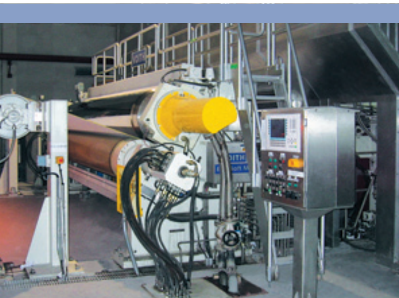
EcoSoft calender installation at Sun Paper, PM 21
