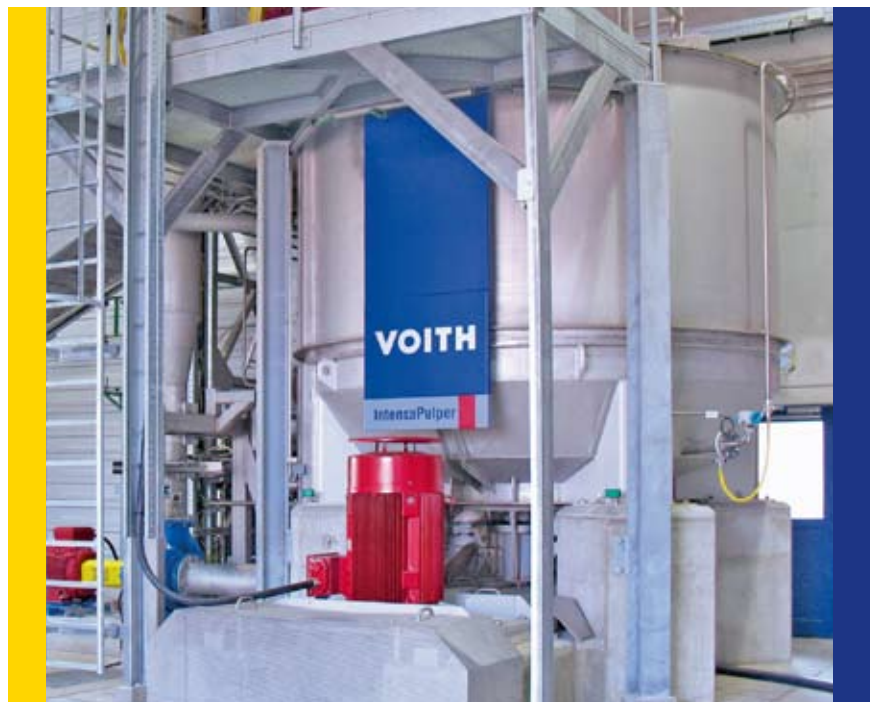
IntensaPulper IP-V in operation.
