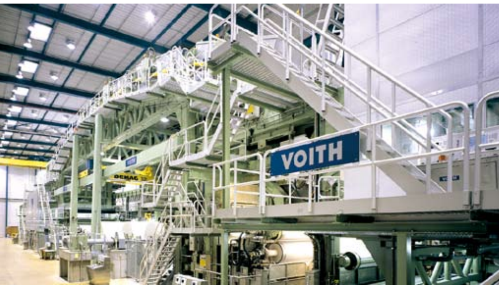
The SM 2 coating machine at the Koehler facilities in Kehl applies the thermo-sensitive coat to the paper.
